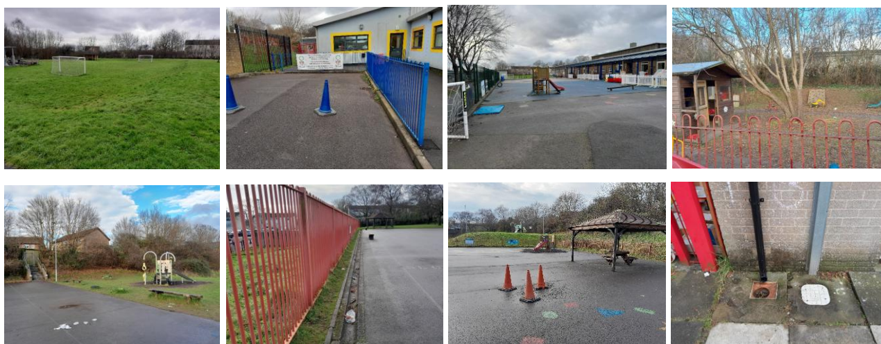
Images of Bryn Celyn & Pen Y Groes' grounds illustrating down pipes and drainage gullies, waterlogged fields and large areas of impermeable ground with ponding
