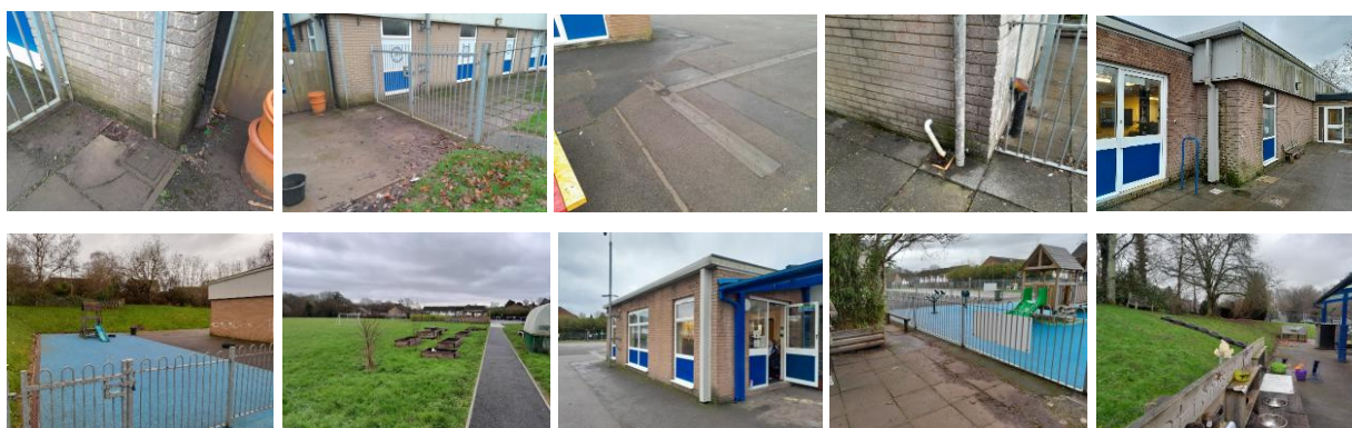
Images of Glyncoed School site illustrating down pipes, drainage gullies, playing fields and areas of impermeable ground with a history of ponding
