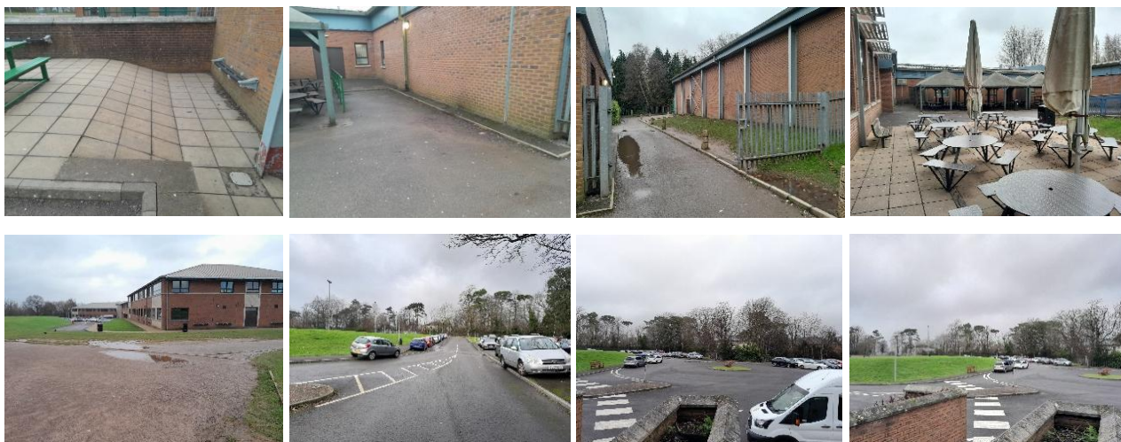
Images of St Illtyd's illustrating down pipes, extensive carparking and areas of impermeable ground with ponding
