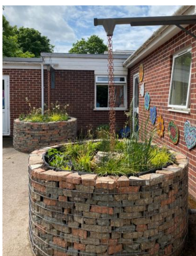
Examples of Disconnected Down pipes and Raised SuDS Planters via Wendy Allen Design
