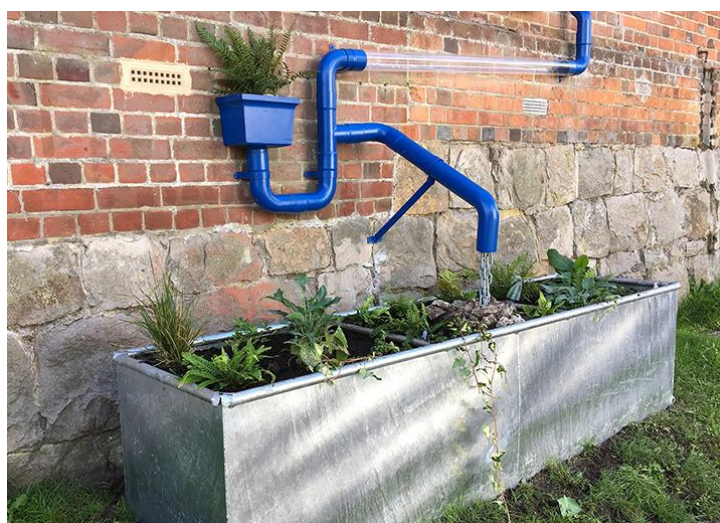
Examples of Disconnected Down pipes and Raised SuDS Planters via Wendy Allen Design
